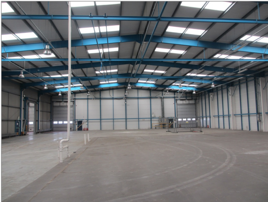
Figure 20: Second cargo hangar interior
