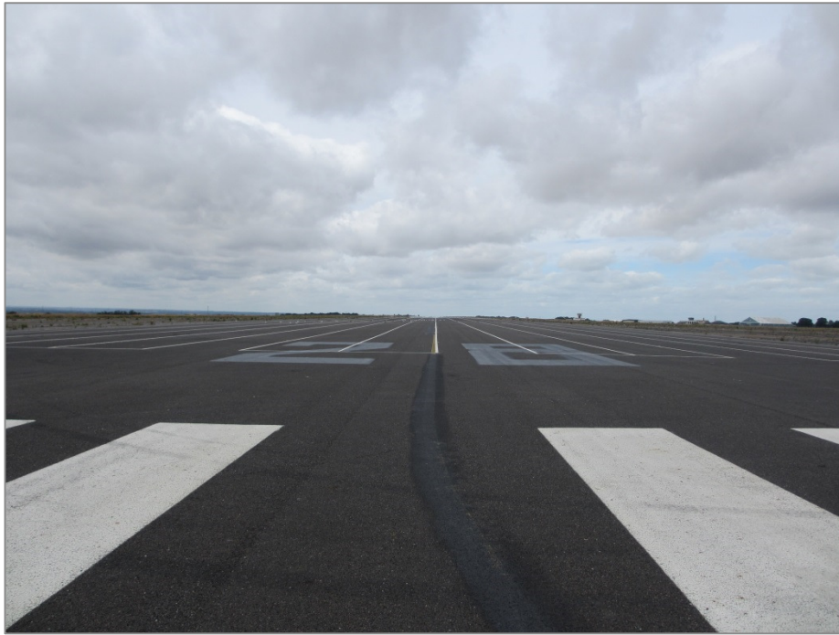
Figure 8: Runway (Rwy) 29 Threshold
