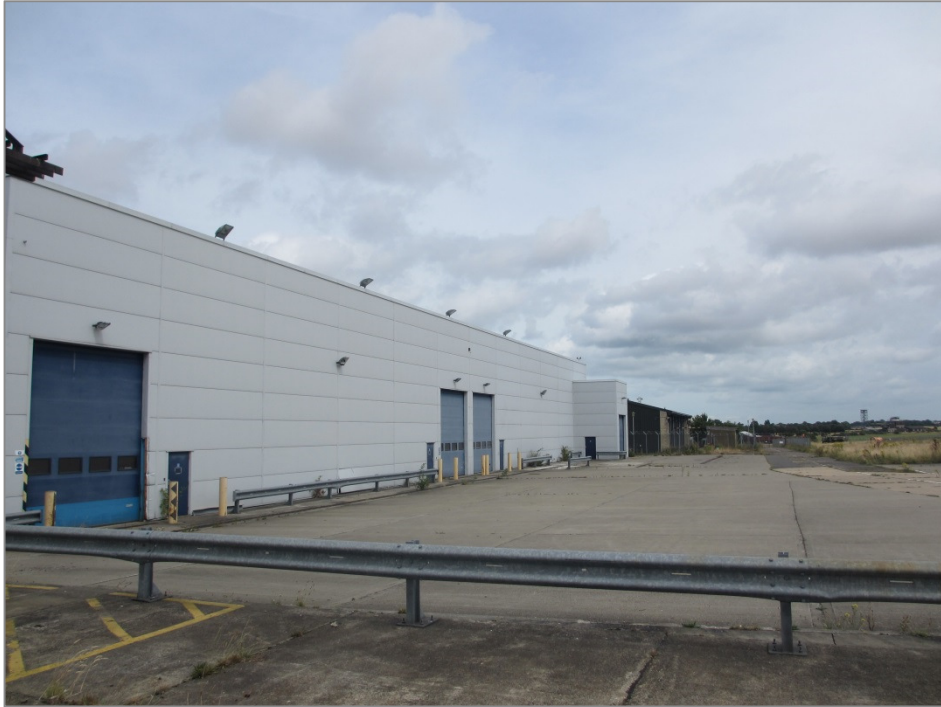
Figure 19: Second cargo hangar exterior
