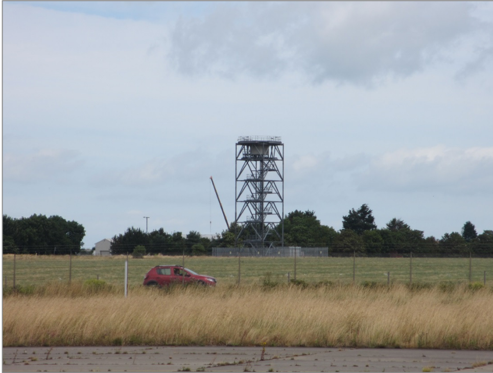
Figure 12: Radar tower with radar removed
