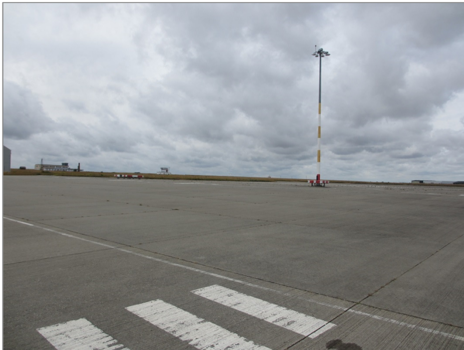
Figure 6: Apron as viewed from terminal
