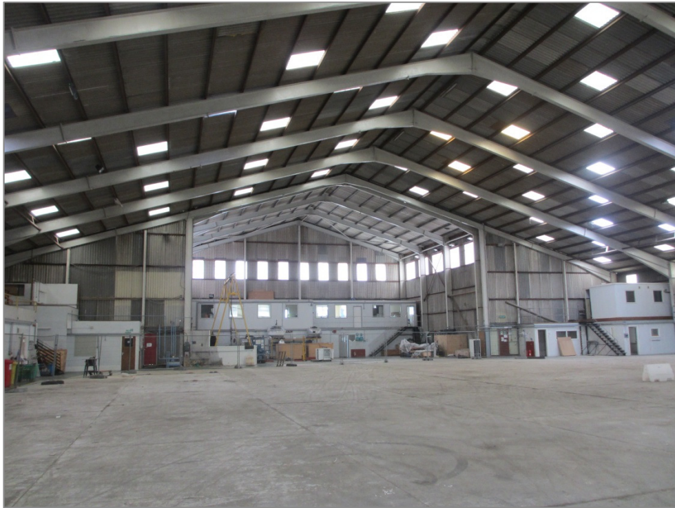
Figure 15: Interior of maintenance hangar
